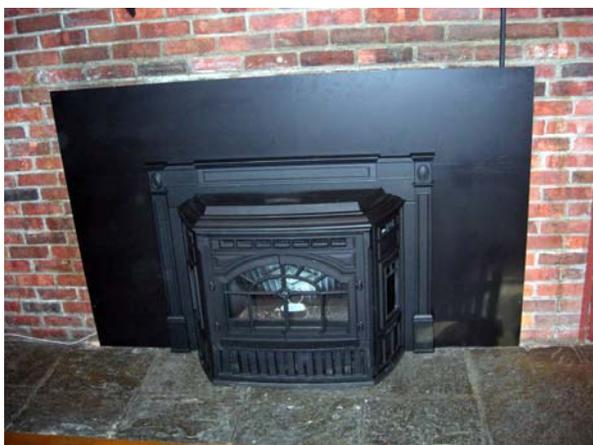
Fig. 1. Quadra-Fire Mt. Vernon AE pellet stove fireplace insert installed at the Big Red Barn, Cornell Univ.
