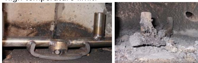
Fig. 2. Fuel-stirring pipe in the burn chamber before and after burning reed canarygrass pellets at a combustion temperature setting of 1600° F. Note melted ash.
