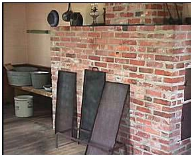
Russian oven in Krause House, photo courtesy of the Mennonite Heritage Museum, Goessel, KS. The metal "zweibach" pans were designed to fit into the long narrow baking chamber. Grass, straw or dried manure served as fuel.
